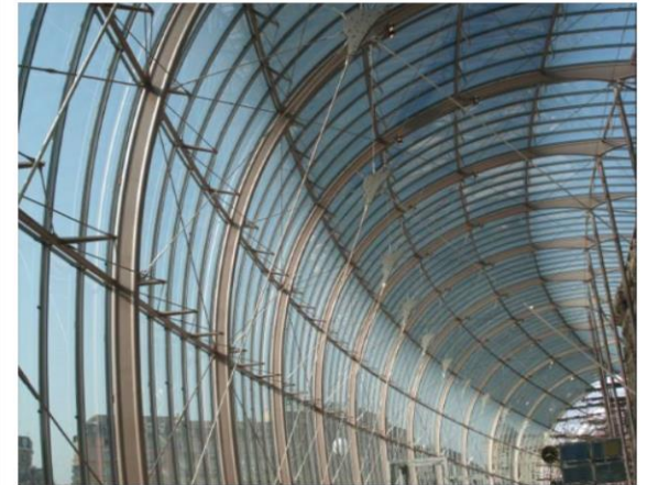
Strasburg Railway Station facade structure 400 tons of steel
