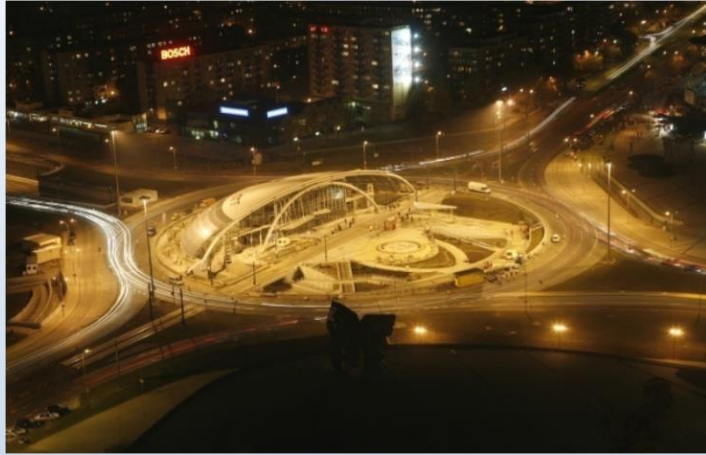
Steel structure cupola over traffic circle in Katowice Poland (240 tons of steel)
