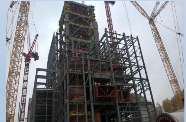
Power Plant Turów 7 000 tons of steel
