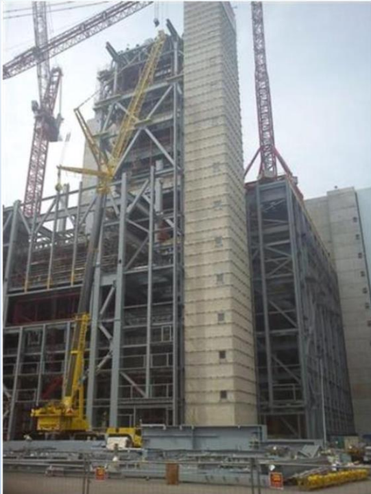
Coal Power Plant Westfalen, Germany 7 793 tons of steel
