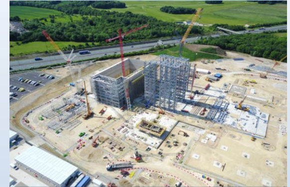
Power Plant Ferrybridge 6 500 tons of steel
