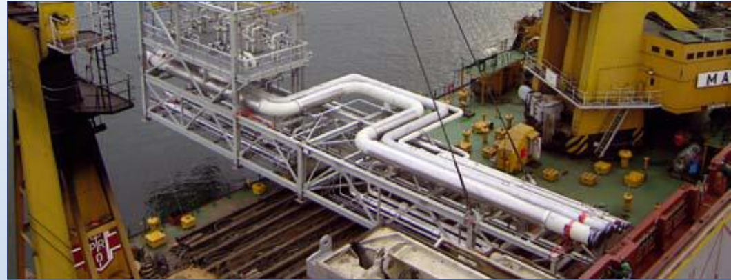
Pipe bridge, Ormen Lange project, Norwegian Sea
