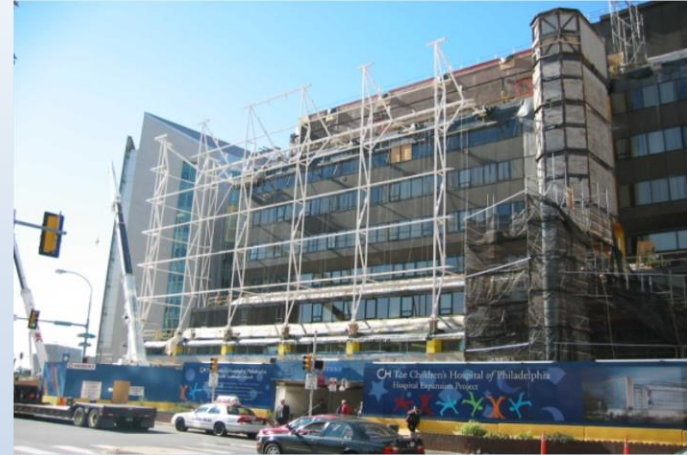
Steel facade at Children's Hospital of Philadelphia, USA (500 tons of steel)
