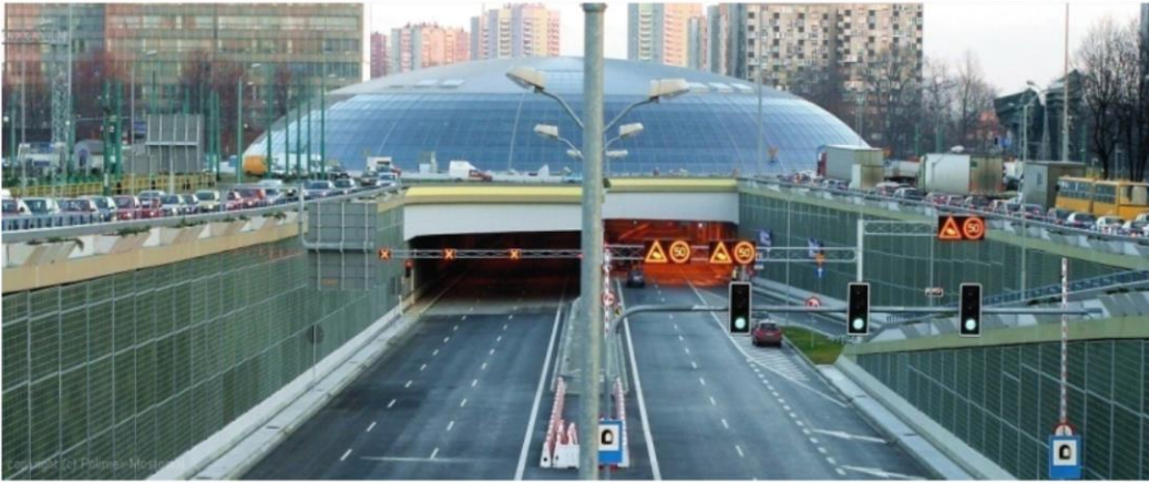
Steel structure cupola over traffic circle in Katowice Polan 240 tons of steel
