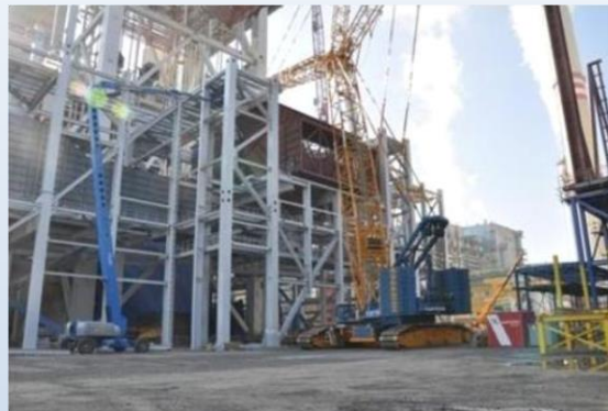
Coal Power Plant Ledvice, Czech Republik 17 270 tons of steel
