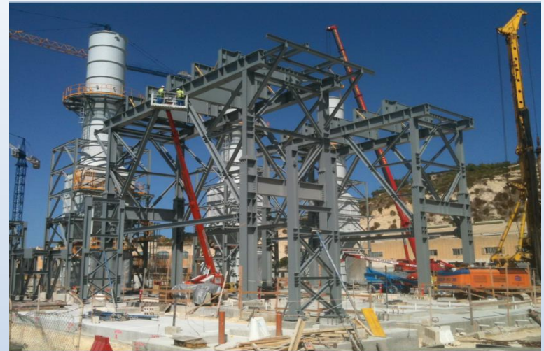
Support structure of the boiler Allborg, Malta 759 tons of steel
