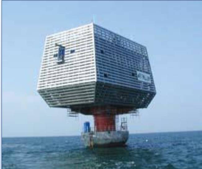
Transformer platform for the Wind Power Plant, Denmark
