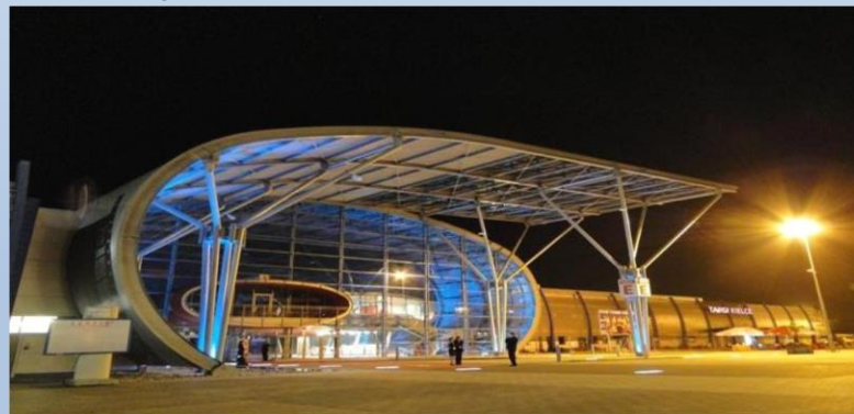
Trade Fair Centre, Exhibition Hall Kielce, Poland (930 tons of steel)
